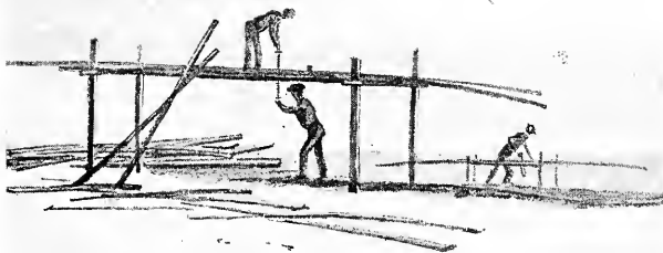
RIPPING TIMBERS FOR THE SCHOONER
